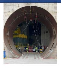
Last month, teams fitted the "Heavy Bridge", which joins together the Reactor Building and Fuel Building on Unit 1. The steel bridge weighing over 12 tonnes enables transfer of equipment into and out of the Reactor Building and protects the Equipment Hatch.
