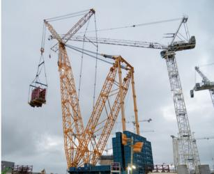
The Reactor Cavity Pool (RCP) was lifted into the Unit 2 Reactor Building, following months of assembly work, welding and concrete pours inside the West Pool Bunker.
