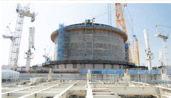
Picture 1: Unit 2's Equipment Hatch successfully positioned, ahead of welding onto Ring Liner 2. The hatch was placed earlier than on Unit 1 after the transferring of learning and experience from one reactor to another.
