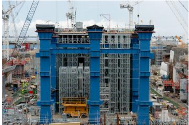
This month spring-boxes have been installed at the top of the columns of the turbine hall ready for the 'table' to be constructed
