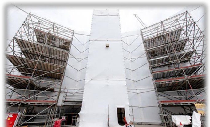
The structure is covered to create a safe working environment
