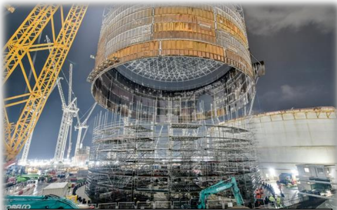
Liner Ring 2 being lifted onto the scaffold structure
