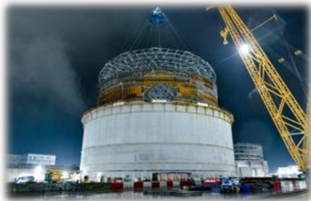
The 308 tonne ring is lifted out of the prefabrication bunker
