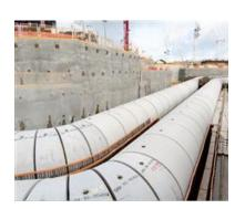
The outlet water pipes for our cooling water system on Reactor 2 have been installed ahead of schedule. These pipes will ferry water between the Pump House and the Turbine Building.
